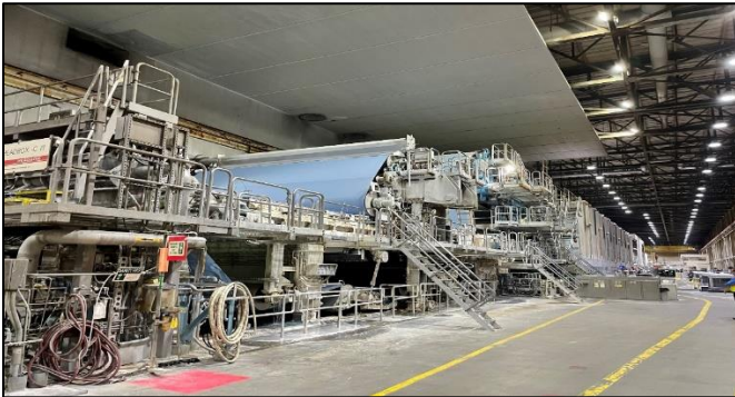
Sappi Skowhegan – Line Rebuild
